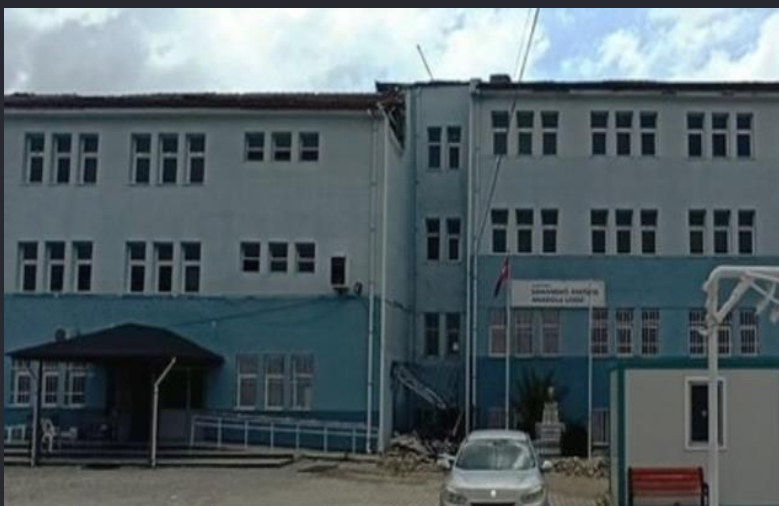
High School repaired.
